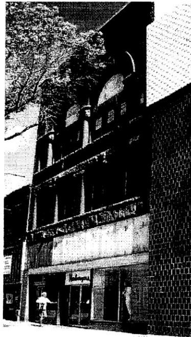
Masonic Temple after removal of screen
