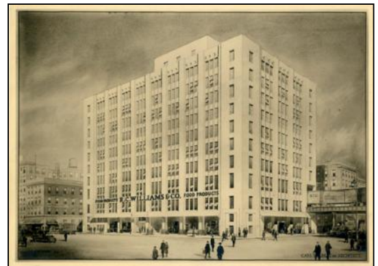
Historic view of R.C. Williams Company Warehouse. Source: Building Conservation Associates
