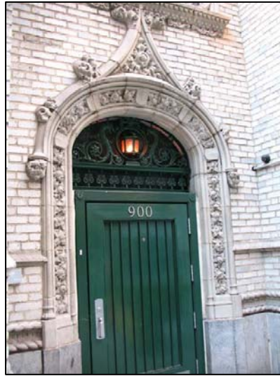
Left: Rodin Studios, 200 West 57 th Street, with Gilbert's ingenious arrangement of double-height studios. Right: Side entrance door at 900 Seventh Avenue. Photos: Marjorie Pearson
