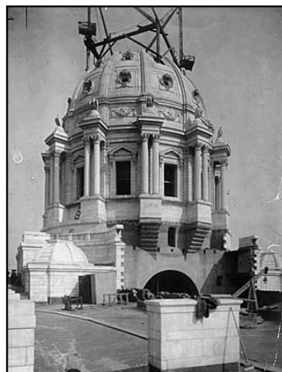
Capitol dome under construction, 1901
